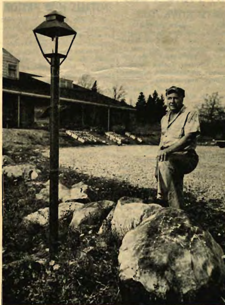
George Wilkinson stands by some foundation stones from John Brown's Richfield tannery. The site of the historic building was uncovered during excavation for the Wilkinson home and market on Route 21.
