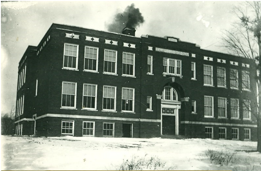
In 1914, Richfield decided to combine all their local schools into one. Richfield Centralized School was opened in 1916. This school was located across from the Richfield United Church of Christ on Streetsboro Road and served the community until 1994. It was first a K-12 school and more classrooms were added in 1934. Another addition as part of the Works Projects Administration which included the auditorium/gymnasium and bus garage. The last graduating class from Richfield High School was in the spring of 1951.
